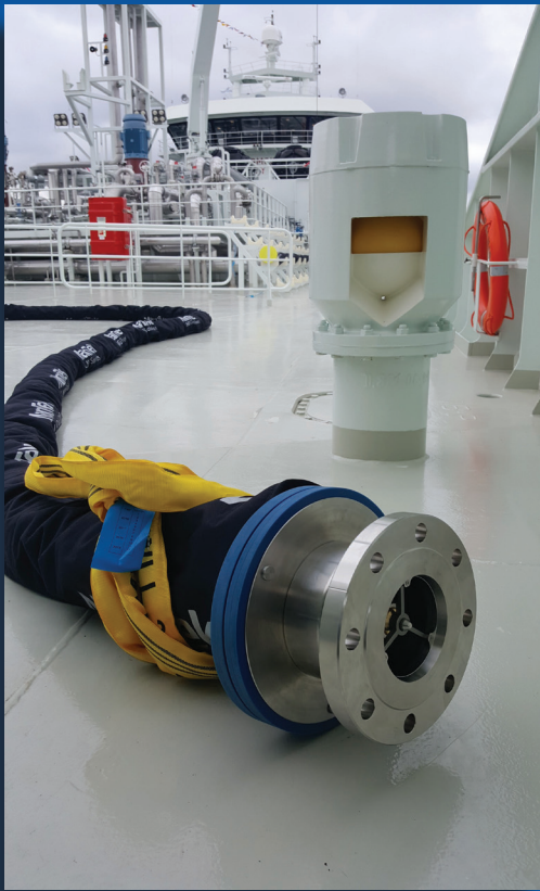
Coralius is fitted with Mann Tek 6-inch PERC and wire drift ESD system.
